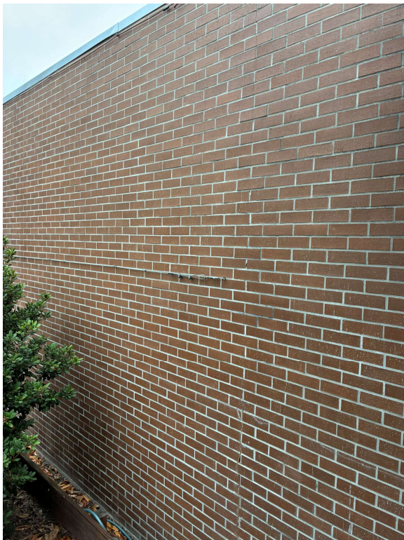
Photo 3 – Exterior Brick Venier
