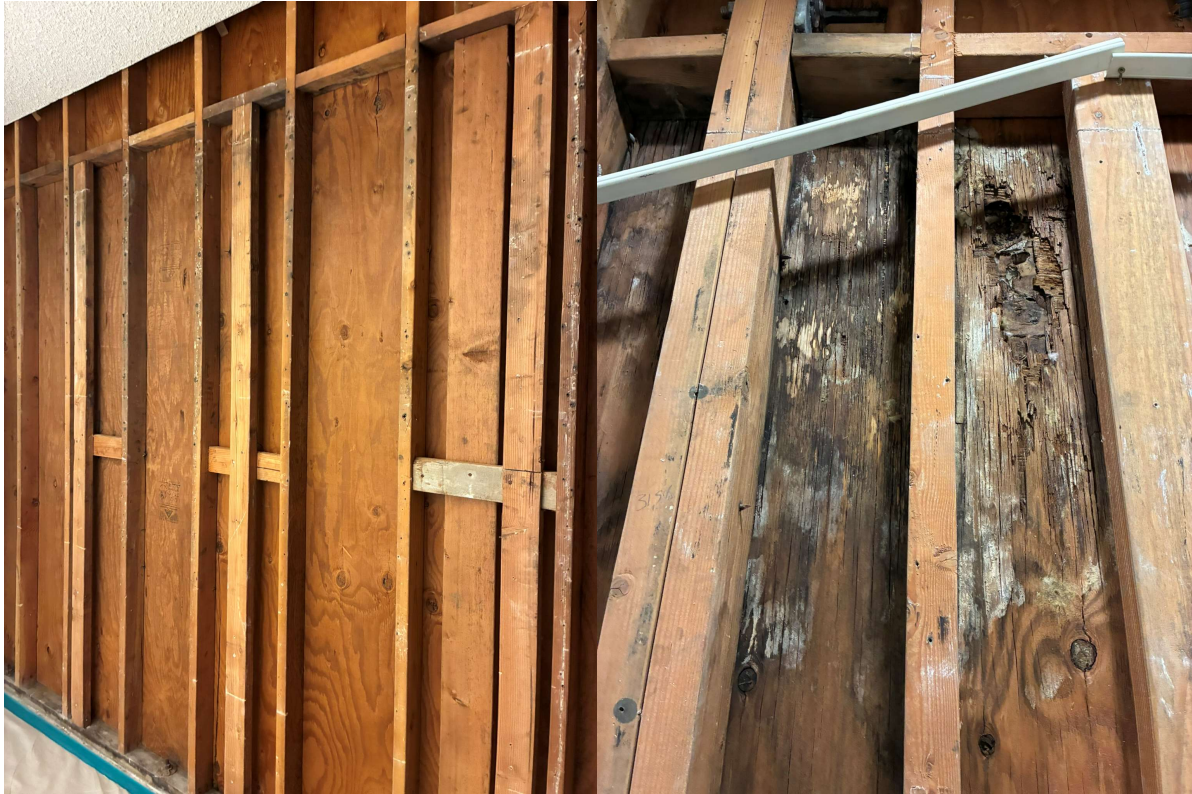
Photo 1 – Interior Wall Cavity
