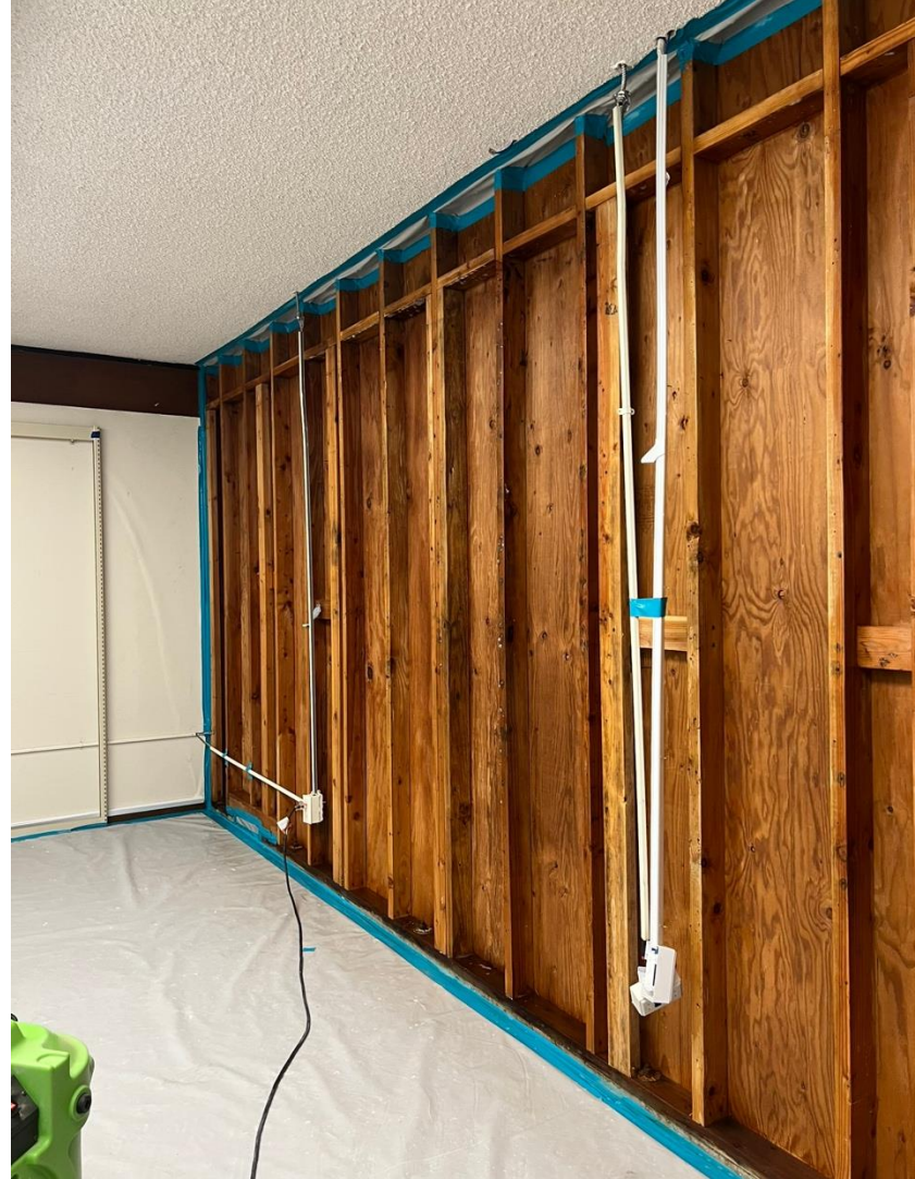
Assessment Structural Damage Exposed on West Exterior Wall
