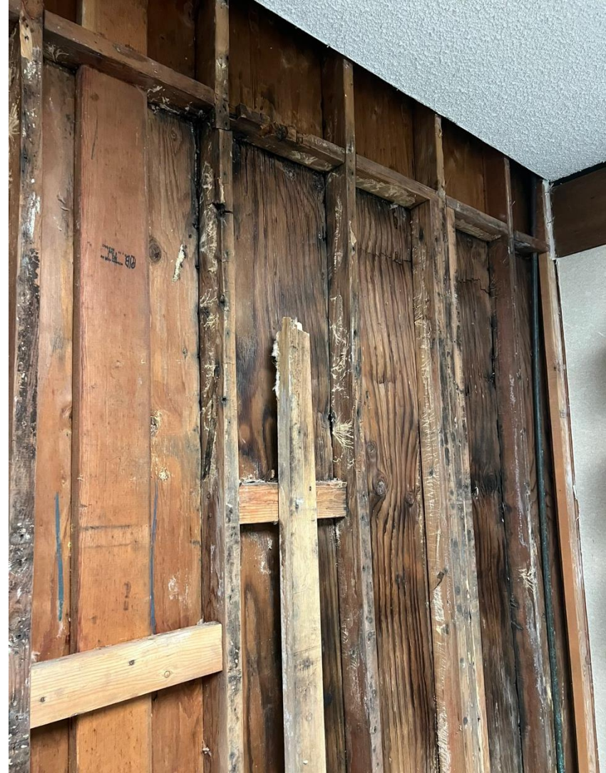
Assessment Structural Damage Exposed on West Exterior Wall
