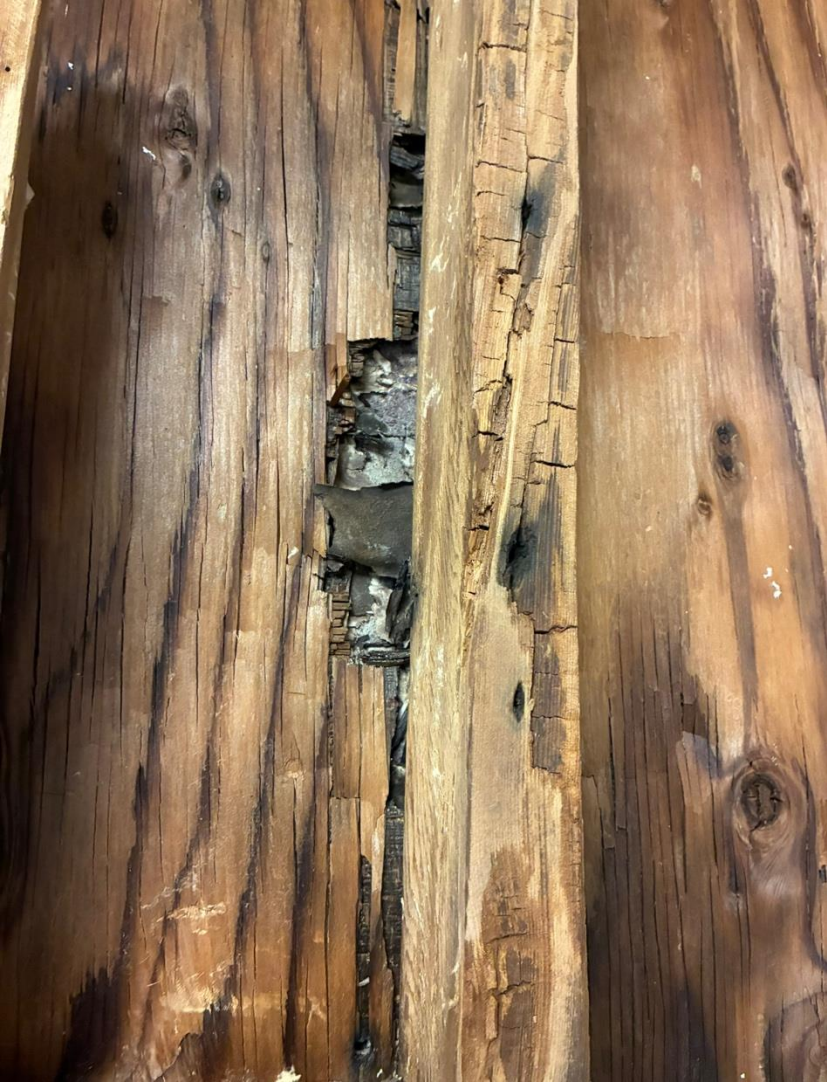
Assessment Structural Damage Exposed on West Exterior Wall
