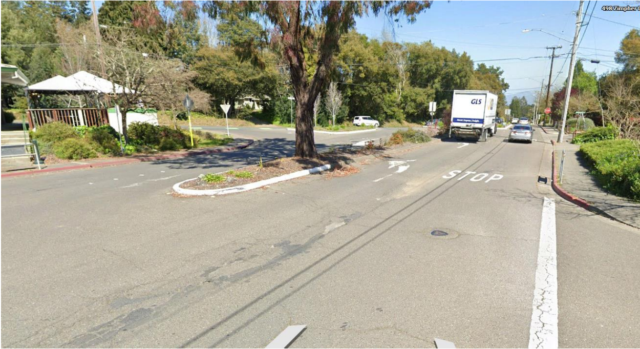
Eastbound travel lanes, east of the pedestrian crossing – 1-block bike lane gap, wide travel lanes encourage higher speeds
