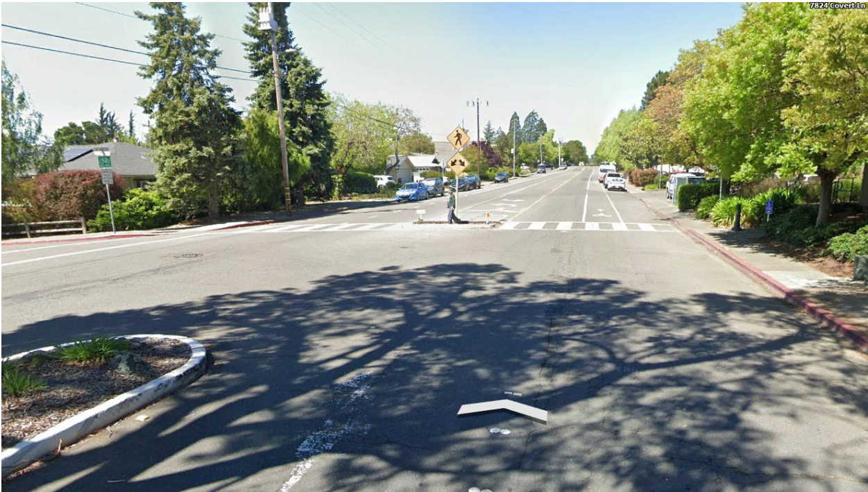
Westbound approach to pedestrian crossing includes through lane and left-turn lane
