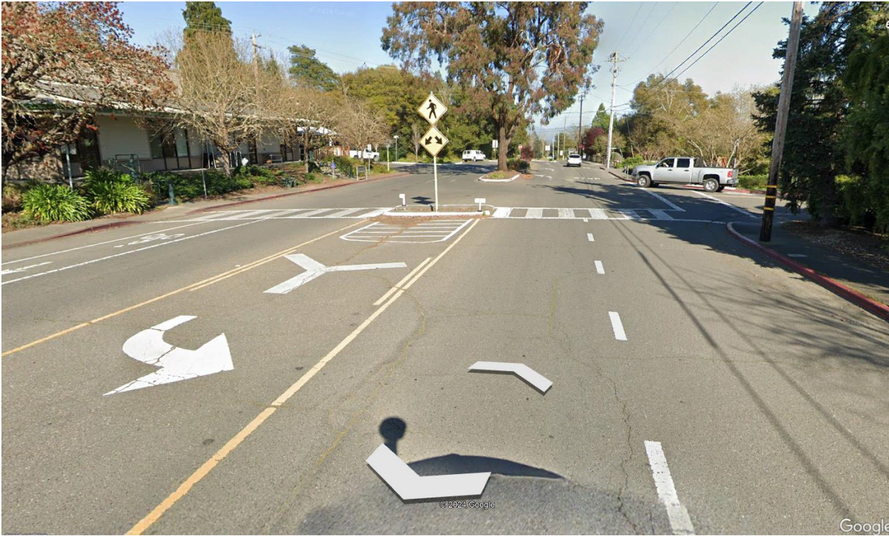
Eastbound approach to pedestrian crossing – end of Covert Lane bike lane creates second travel lane, increasing pedestrian exposure to vehicle traffic
