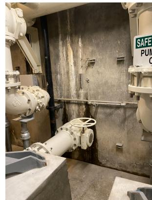
**DESCRIPTION:** Install a liner or protective coating to the wet well. An initial assessment of the wet well concluded that the epoxy filler in the wet well is failing and is leaking. Making the repair will extend the lifespan of the wet well to keep it in operation.
