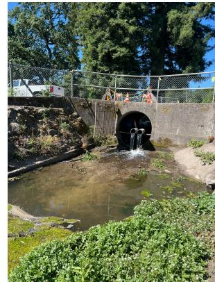
**DESCRIPTION:** Trenchless repair of the 60-inch corrugated metal storm drain pipe.
