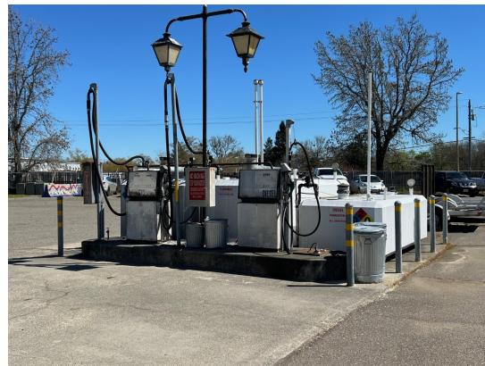
**DESCRIPTION:** Upgrade the filling station to meet new Air Resources Board (CARB) requirements. The project includes replacement of pumps with vapor capture system, monitoring system, and site lighting.
