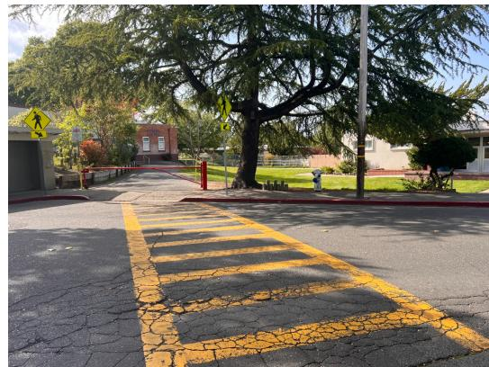
**DESCRIPTION:** Taft Street/Sunset Avenue – upgrade crosswalk markings including advanced yield markings and install double-sided flashing pedestrian crossing signs with circular LED beacons in similar style to other Sebastopol crossings. Install advanced pedestrian crossing signage. Upgrade curb ramps to comply with current ADA standards. Install edge line striping for traffic calming on Sunset Avenue between Taft Street and Johnson Street.
