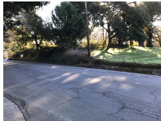
**DESCRIPTION:** Phase 2 is for installing bike lanes and repaving Bodega Avenue from Robinson Rd./Nelson Way to Pleasant Hill Road. Due to funding constraints, this project was split into two phases with Phase 1 being High Street to Robinson/Nelson and Phase 2 continuing on to Pleasant Hill Road. Due to the extremely poor condition of the road in this Phase 2 section, the roadbed will need to be reconstructed rather than overlayed.
