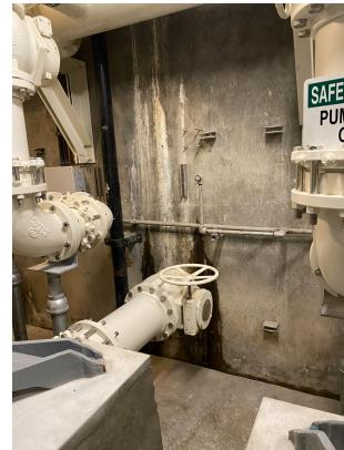
**DESCRIPTION:** Install a liner or protective coating to the wet well. An initial assessment of the wet well concluded that the epoxy liner in the wet well is failing and is leaking. Making the repair will extend the lifespan of the wet well to keep it in operation.
