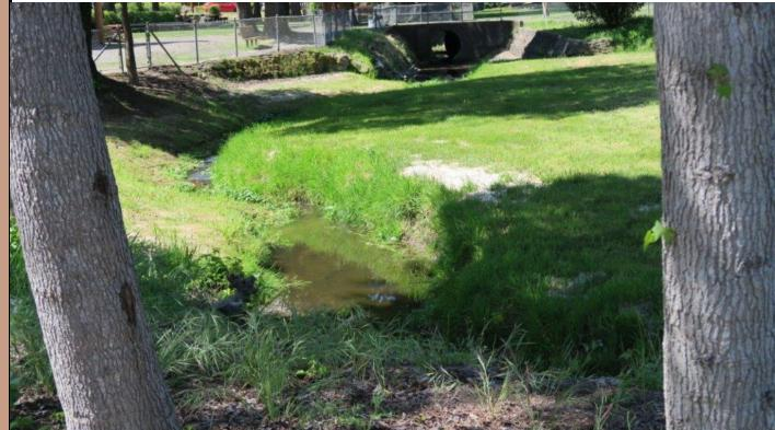
**DESCRIPTION:** This project is a multi-year effort including a Maintenance Study to identify the maintenance activities for the storm drain and outfall, priorities, and estimated costs. This segment of Calder Creek pipeline is filled with silt and debris and needs to be "dredged" out to maintain hydraulic capacity.
