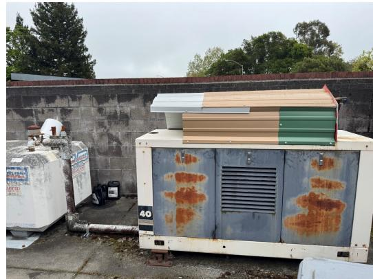
**DESCRIPTION:** Replacement and upgrade of existing 40kW emergency generator to a new generator that will support the EOC, dispatch room, and other essential emergency support services at the Police Station.
