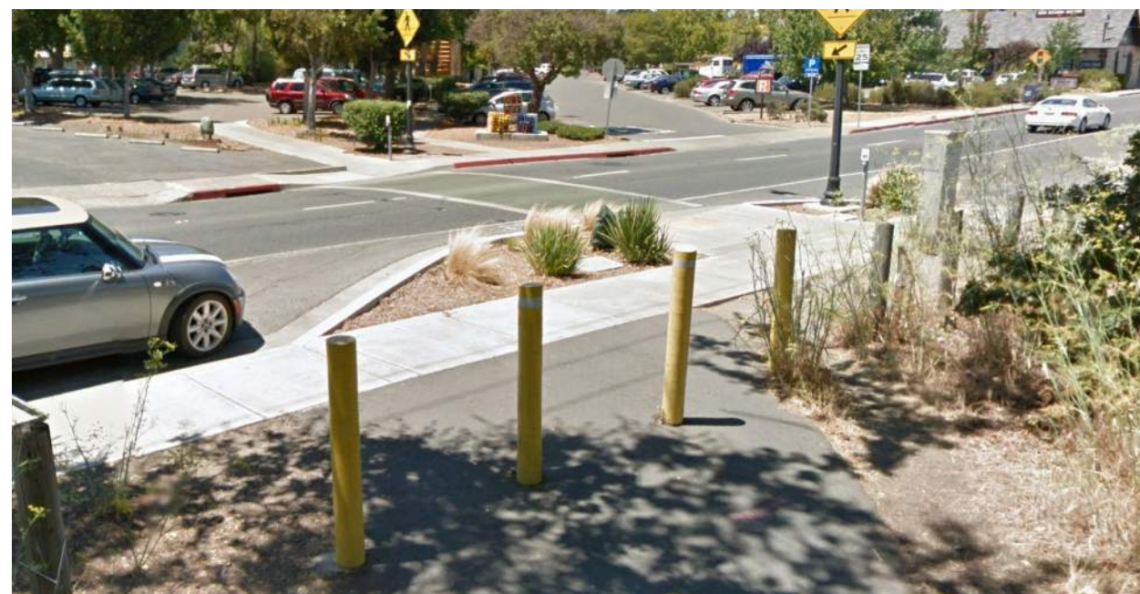
Existing terminus of the Joe Rodota Trail, looking west
