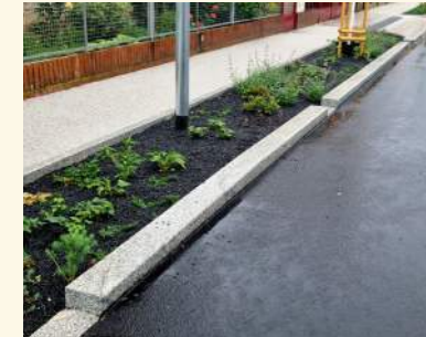
vegetated sidewalk extension
