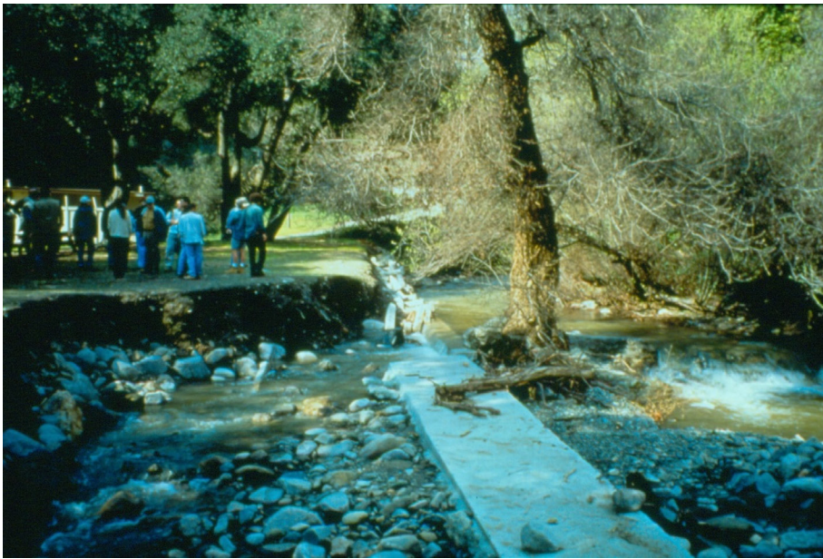
Photo 1: Meander removal to straighten stream resulted in stream meandering around grade control structure.
