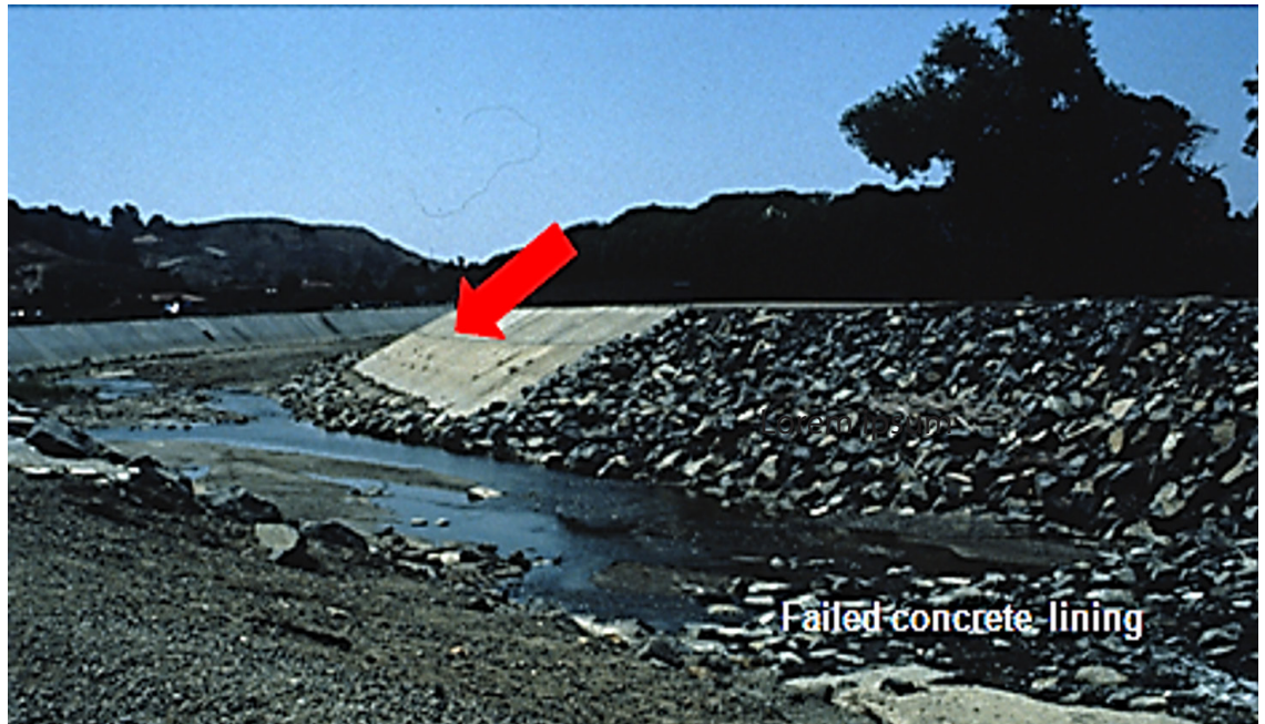
Photo 2: Failed concrete lining due to incision and incorrect channel geometry.
