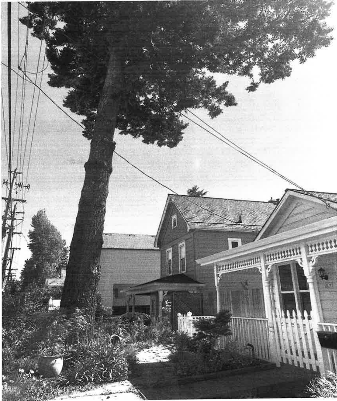
Photo provided by insured showing the subject tree in close proximity to the residence and utility lines.
