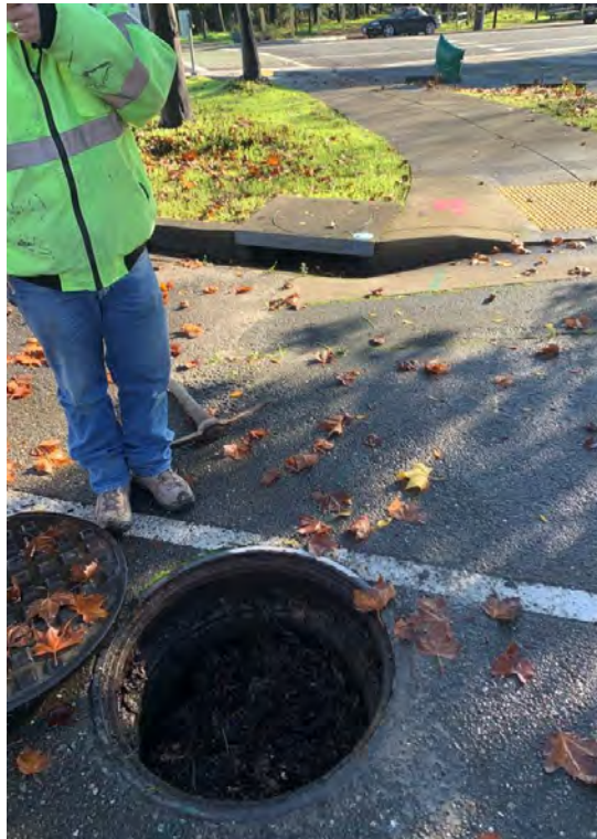
Figure 5 GHD staff at a manhole upstream from Petaluma Ave. with sediment accumulation at the manhole rim along the southern run of Reach 3 along a run of 6'x3' arched concrete conduit.
