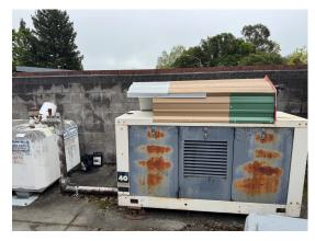
**DESCRIPTION:** Replacement and upgrade of existing 40kW emergency generator to a new generator that will support the EOC, dispatch room, and other essential emergency support services at the Police Station.
