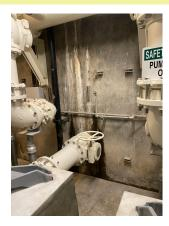
**DESCRIPTION:** Install a liner or protective coating to the wet well. An initial assessment of the wet well concluded that the epoxy filler in the wet well is failing and is leaking. Making the repair will extend the lifespan of the wet well to keep it in operation.
