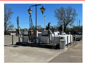
**DESCRIPTION:** Upgrade the filling station to meet new Air Resources Board (CARB) requirements. The project includes replacement of pumps with vapor capture system, monitoring system, and site lighting.
