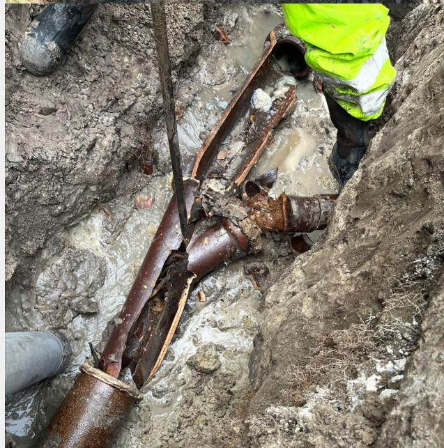
Clay sewer piper, failed connection joint tree root intrusion blockage
