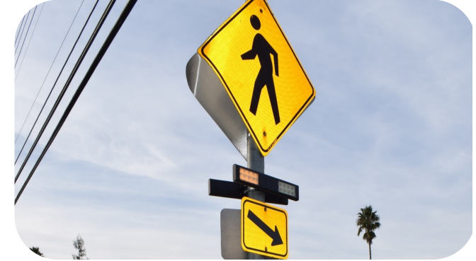
Rectangular Rapid Flashing Beacon
