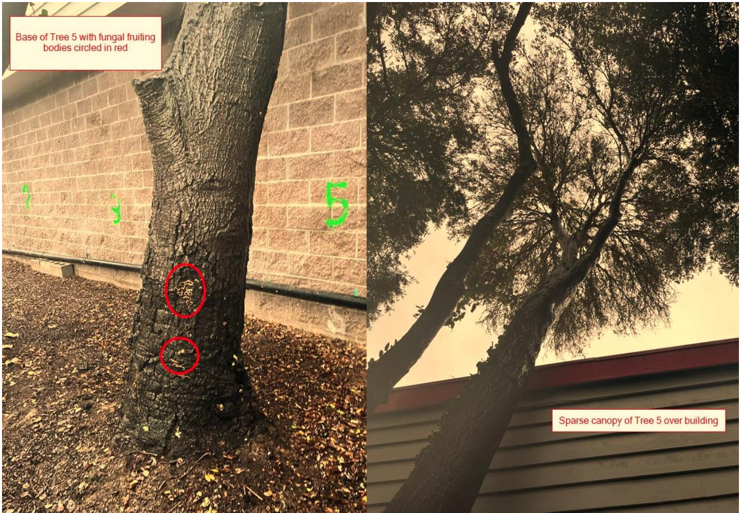
Figure 4. Decaying trunk and sparse canopy of Tree 5.
