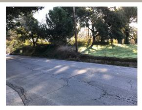
**DESCRIPTION:** Phase 2 is for installing bike lanes and repaving Bodega Avenue from Robinson Rd./Nelson Way to Pleasant Hill Road. Due to funding constraints, this project was split into two phases with Phase 1 being High Street to Robinson/Nelson and Phase 2 continuing on to Pleasant Hill Road. Due to the extremely poor condition of the road in this Phase 2 section, the roadbed will need to be reconstructed rather than overlayed.
