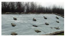
the slope, sandbags are placed around the perimeter with additional bags placed randomly for weight. If the slope is steep, wooden stakes can be driven into the ground just above the area to be protected. The stakes are 4 feet apart with a 1-foot stagger. The plastic is secured to the stakes with tie-down buttons or small round rocks (see Figure 13).
