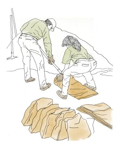
Figure 1: Proper sandbag filling
