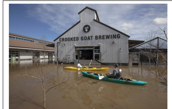
In February 2019, several businesses in The Barlow shopping district suffered from flooding after an atmospheric river stalled over the Russian River Watershed. An estimated two-thirds of the shopping district was flooded, including Park Village, a City-owned low income housing site, and the Community Cultural Center located on Morris Street. Photo Credit: John Burgess/The Press Democrat
