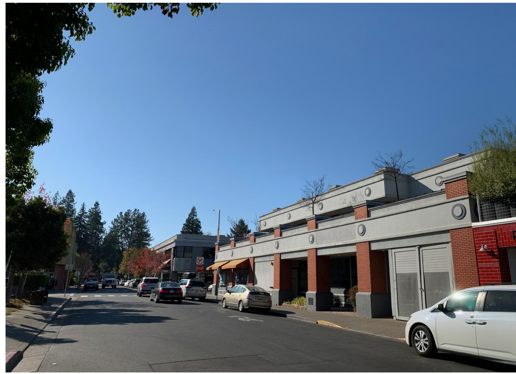
1 FROM BURNETT STREET LOOKING WEST TOWARD SOUTH MAIN #2
