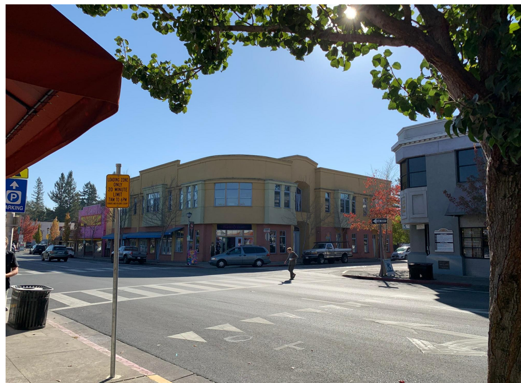
9 FROM PROJECT ENTRY LOOKING SOUTH WEST ACROSS S. MAIN
