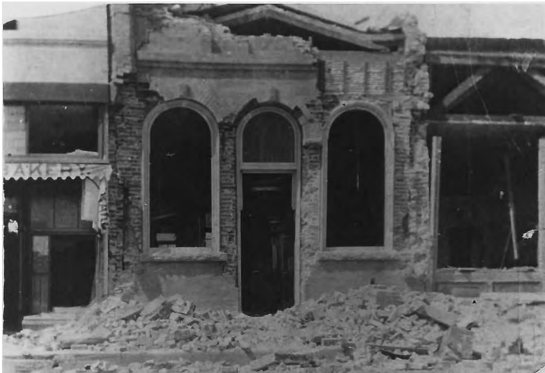
Figure 10: Photograph of the damage to the Bank of Sebastopol (no longer extant) on Main Street near Bodega Avenue caused by the 1906 earthquake (Courtesy of the Sonoma County Library).
