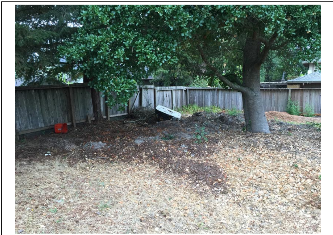
Photo 6: View of northwest corner of property of debris and soil piles.
