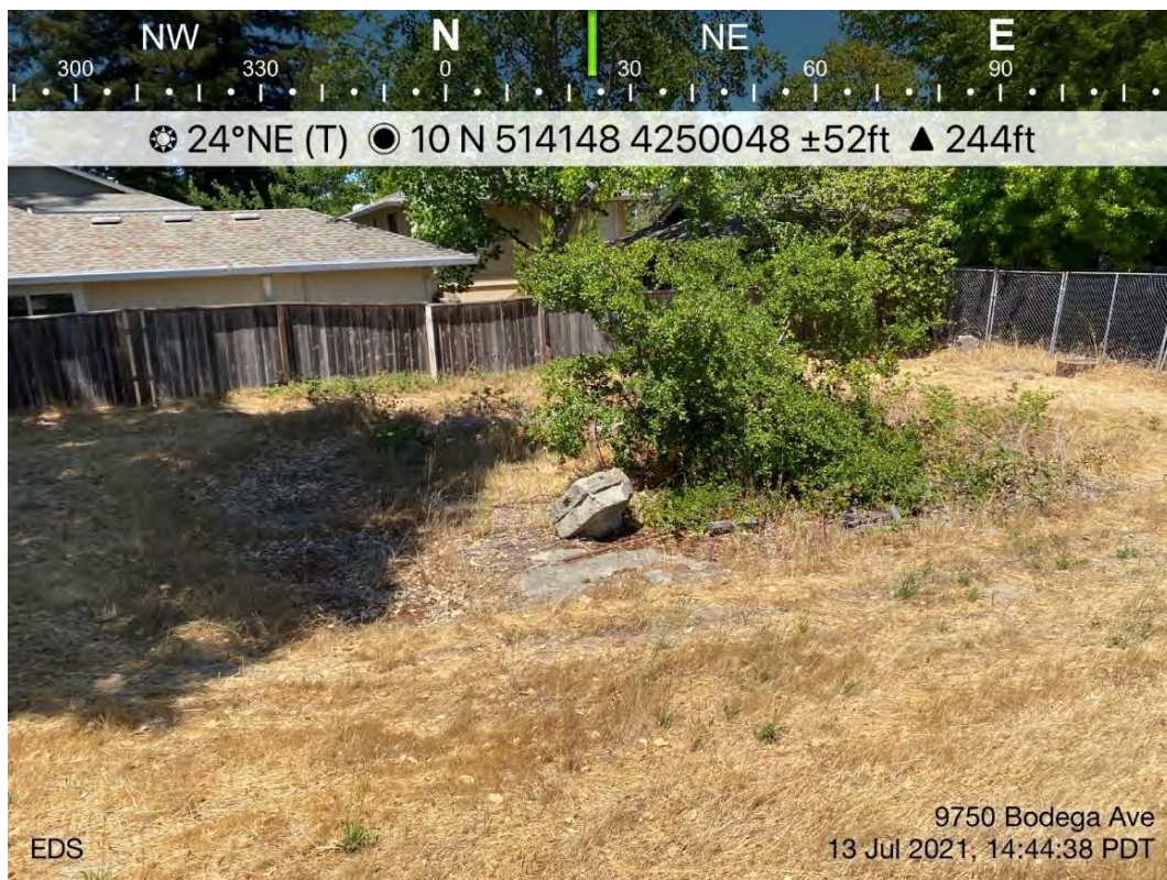
Figure 28: Overview of the foundation and construction materials observed in the northern portion of the Project Area, facing north/northwest.
