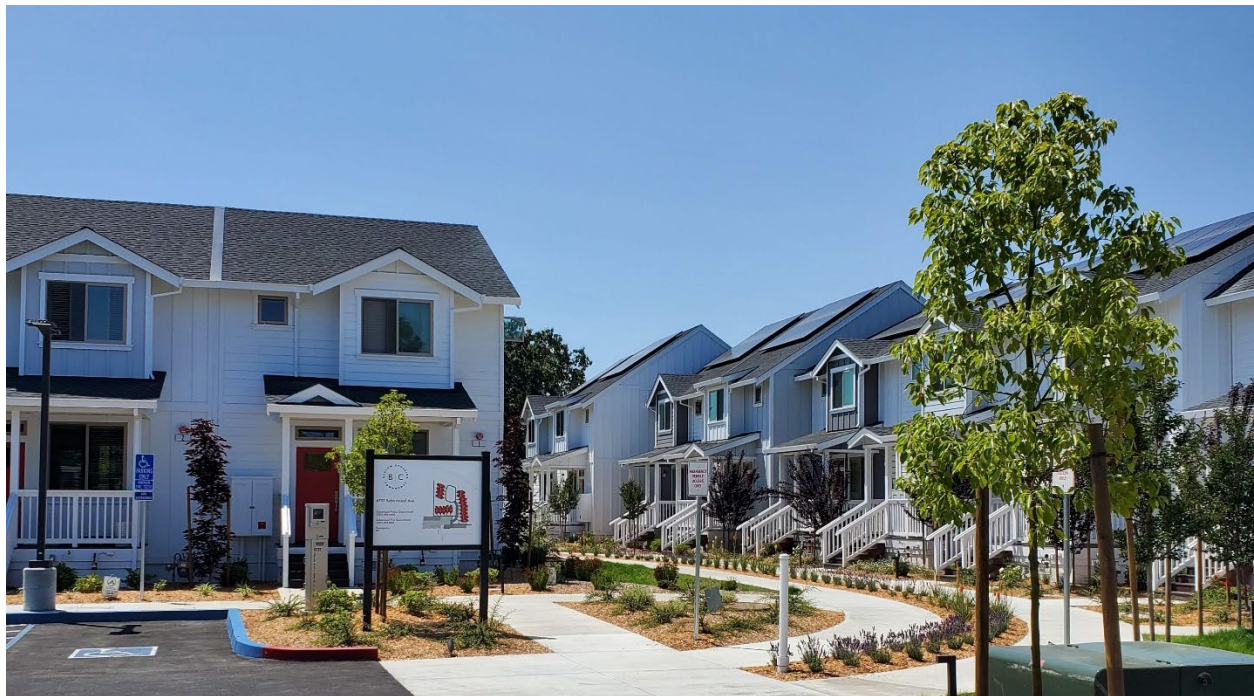
Figure 19: Barlow Crossings Townhomes
