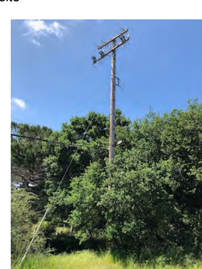
18 Power pole @ front of site
