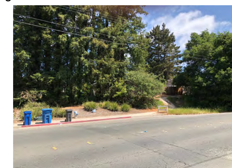
19 Street frontage & end of sidewalk at 7990 Bodega Ave.
