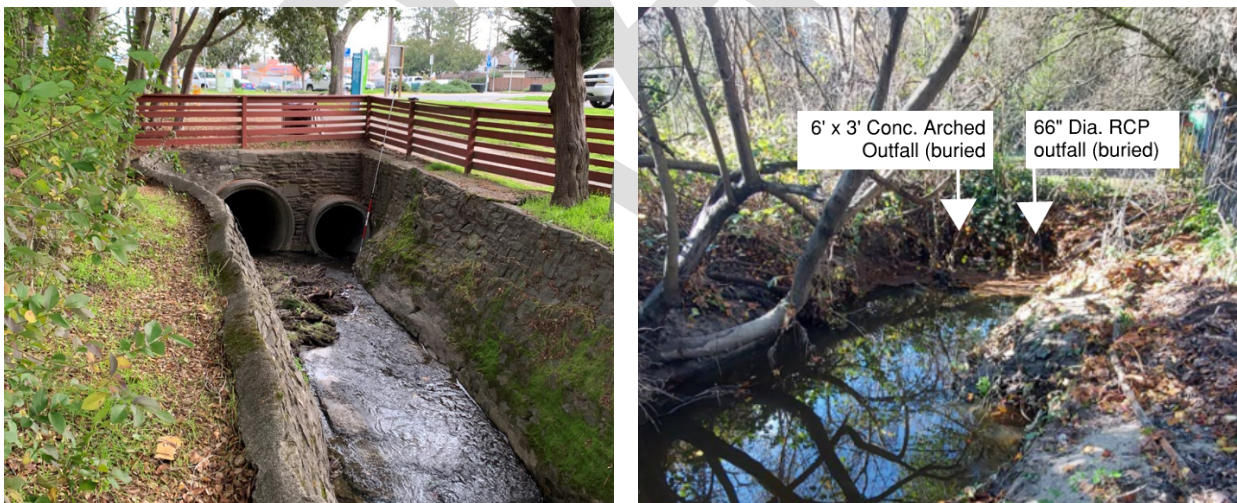
Figure 4: Left: Calder Creek at downstream end of Ives Park at the inlet of the parallel, underground pipes. Right: Calder Creek outfalls at the Laguna De Santa Rosa floodplain.
