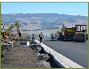
University District Development: Asphalt Paving Operations for New Street Construction.
