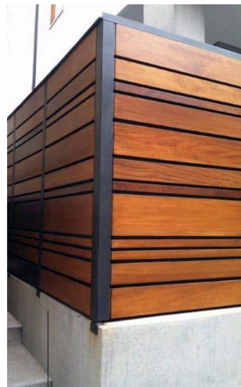
5' TALL PRIVACY FENCE WITH HORIZONTAL WOOD BOARD AND STEEL POST ON RETAINING WALL - CLEAR REDWOOD
