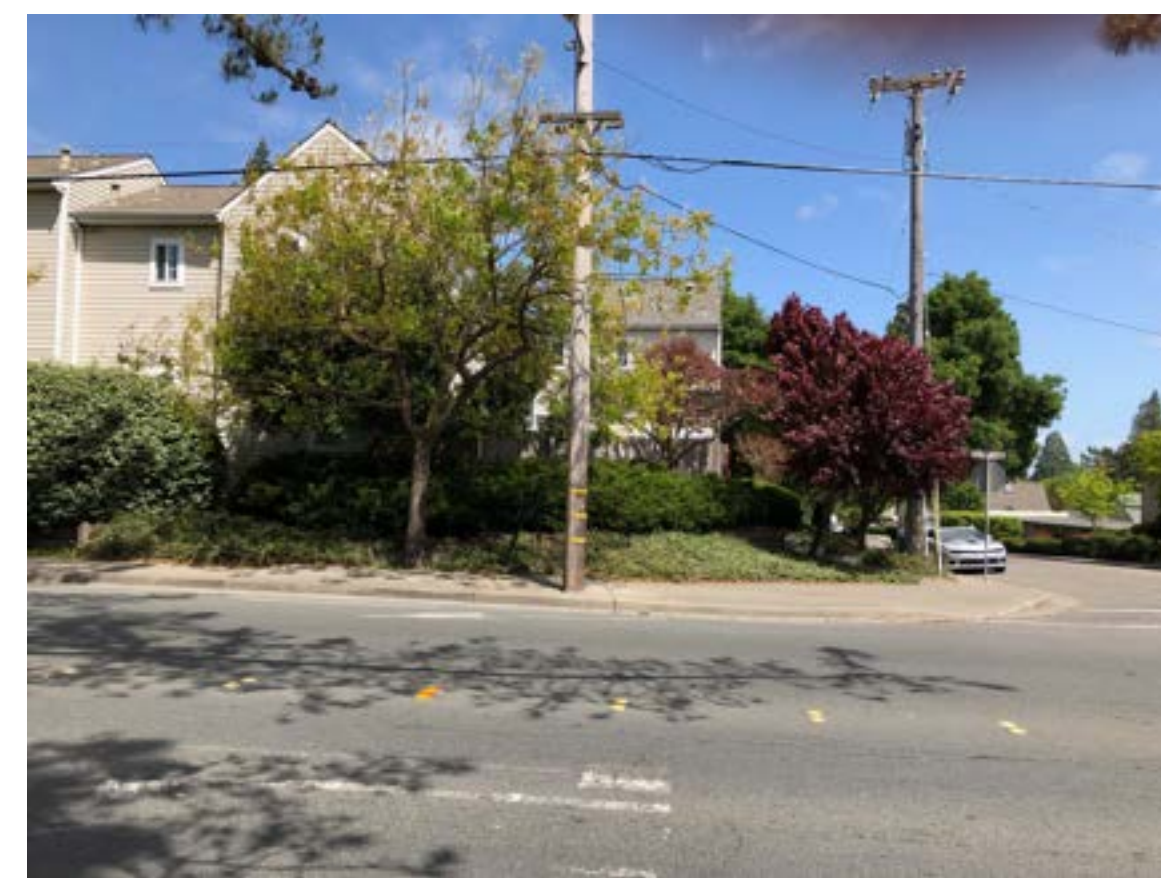
3 Looking north along east side of 120-132 Golden Ridge Ave.
