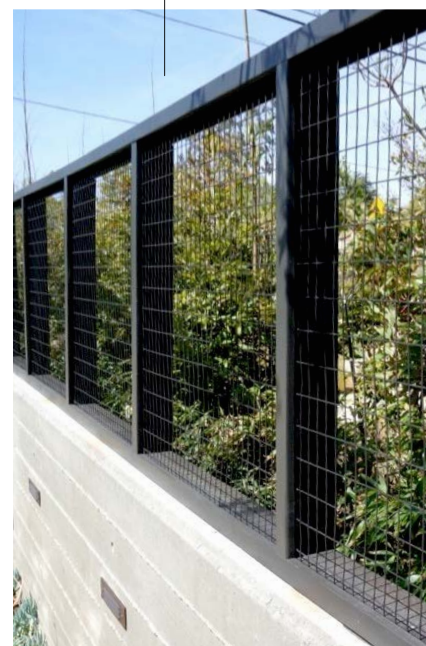
42" TALL HOG WIRE FENCE WITH POWDER-COATED STEEL PANELS ON 2x12 HORIZONTAL ROUGH SAWN BOARD FORM CONCRETE RETAINING WALL
