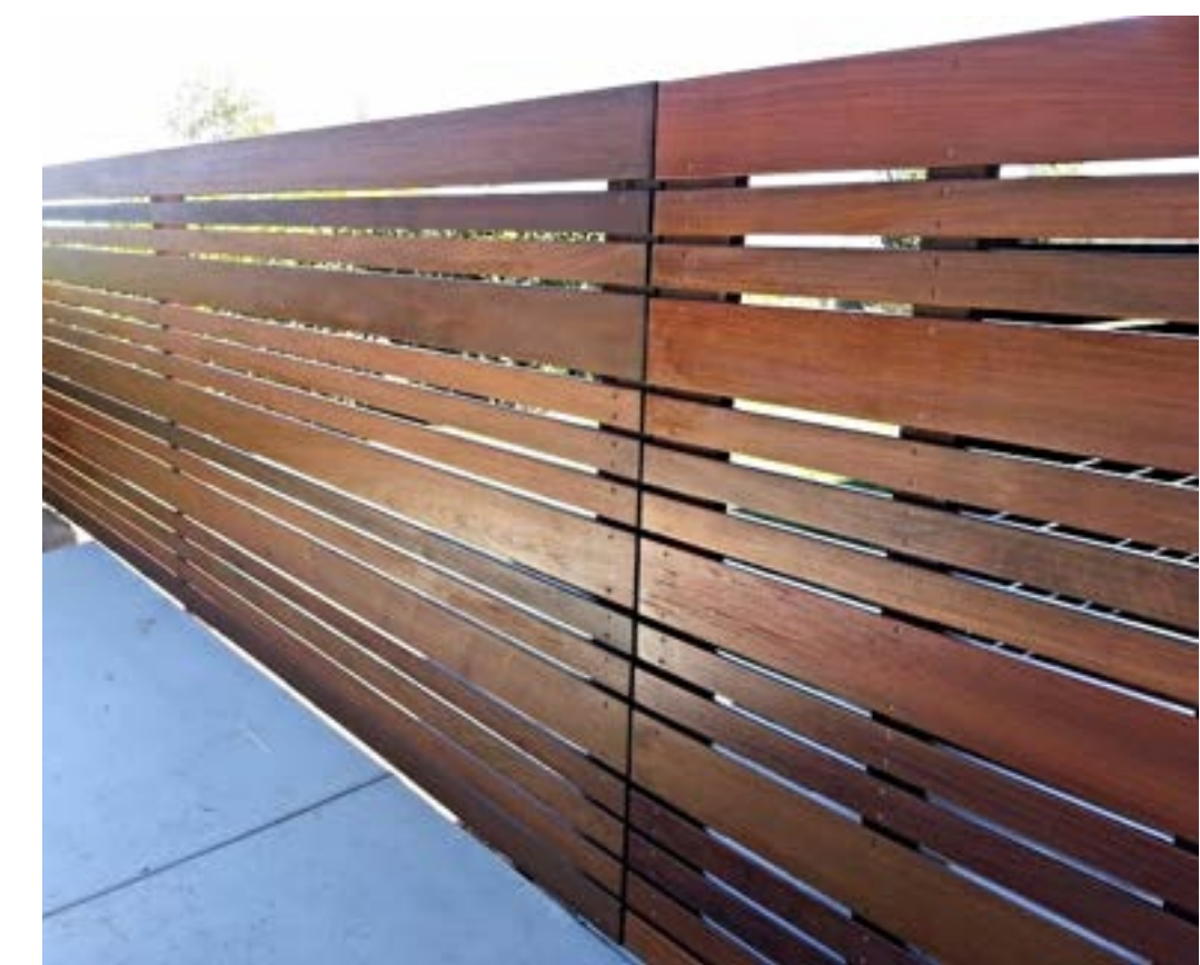
5' TALL PRIVACY FENCE WITH HORIZONTAL WOOD BOARD AND STEEL POST ON RETAINING WALL - CLEAR REDWOOD
